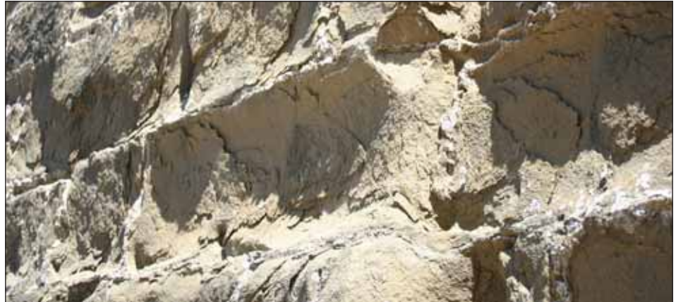
A close-up of sandstone blocks at the pumphouse chimney base showing the extreme flaking and flaking of the sandstone blocks that results from their significant clay content. Image: © K A Rodgers 2005
