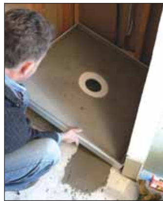
Above: Installing the shower tray onto an existing floor.
