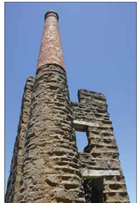
Kawau's 19th Century copper mine pumphouse chimney. The severe weathering of the Mahurangi sandstone blocks at the chimney's base contrast with the brick of the chimney's upper stack. Image: © K A Rodgers 2005
