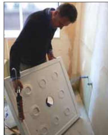
Right: The 100% waterproof shower tray underside showing support rings for secure placement onto an existing concrete or timber floor.
